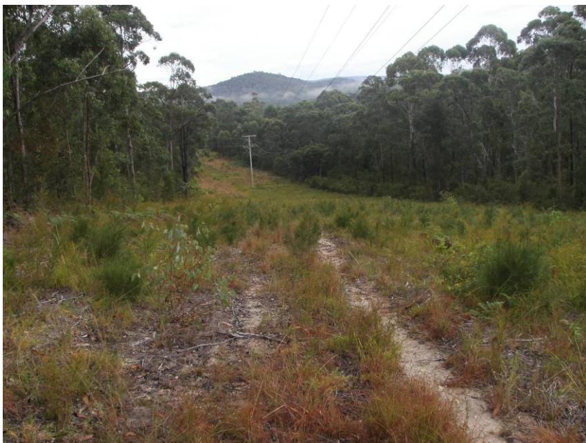
Plate 12: SU3 showing slashed area along north trending power line easement with dirt access track and erosion scalds along - view to north.
