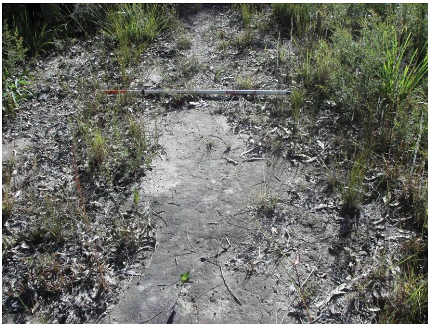
Plate 18: SU4 showing erosion scald at break of slope to south of Frys Creek.
