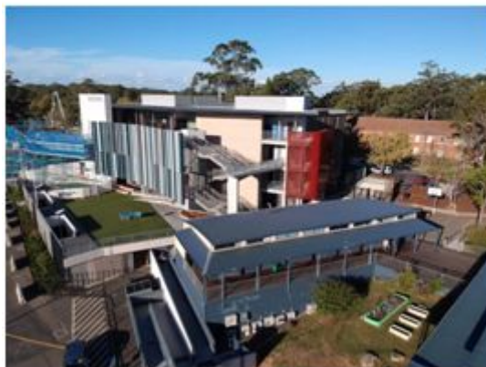
Image 1: SW corner unit in Block A, at sixth floor window. Six metre set back from School boundary (fence line).
