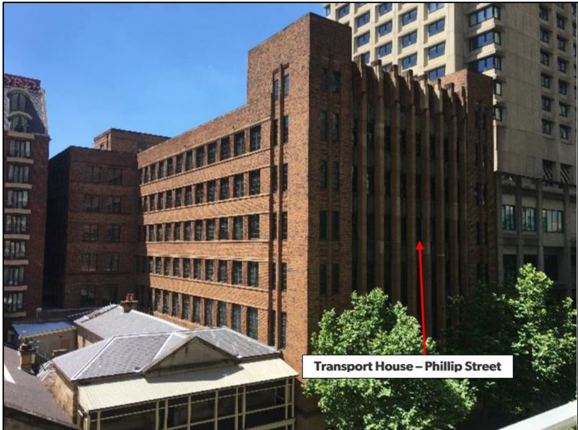
Figure 5 – Phillip Street (western) elevation of Transport House (Source: Department's AR)
