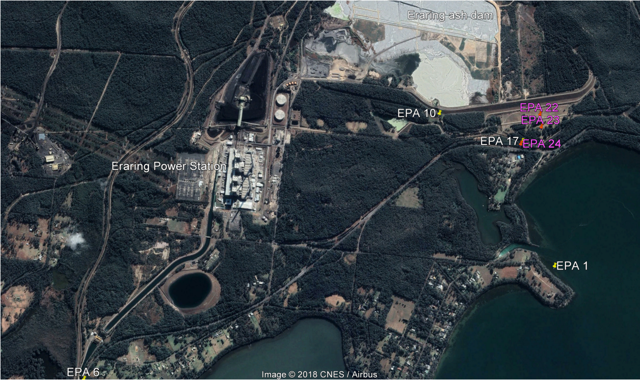
Figure 11: Eraring power station EPL surface water and groundwater monitoring points for which monthly data is made public
