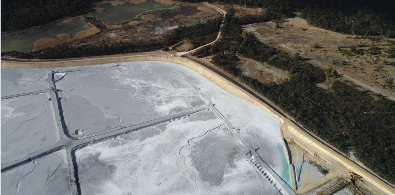
Eraring ash dam cells made from ash.
