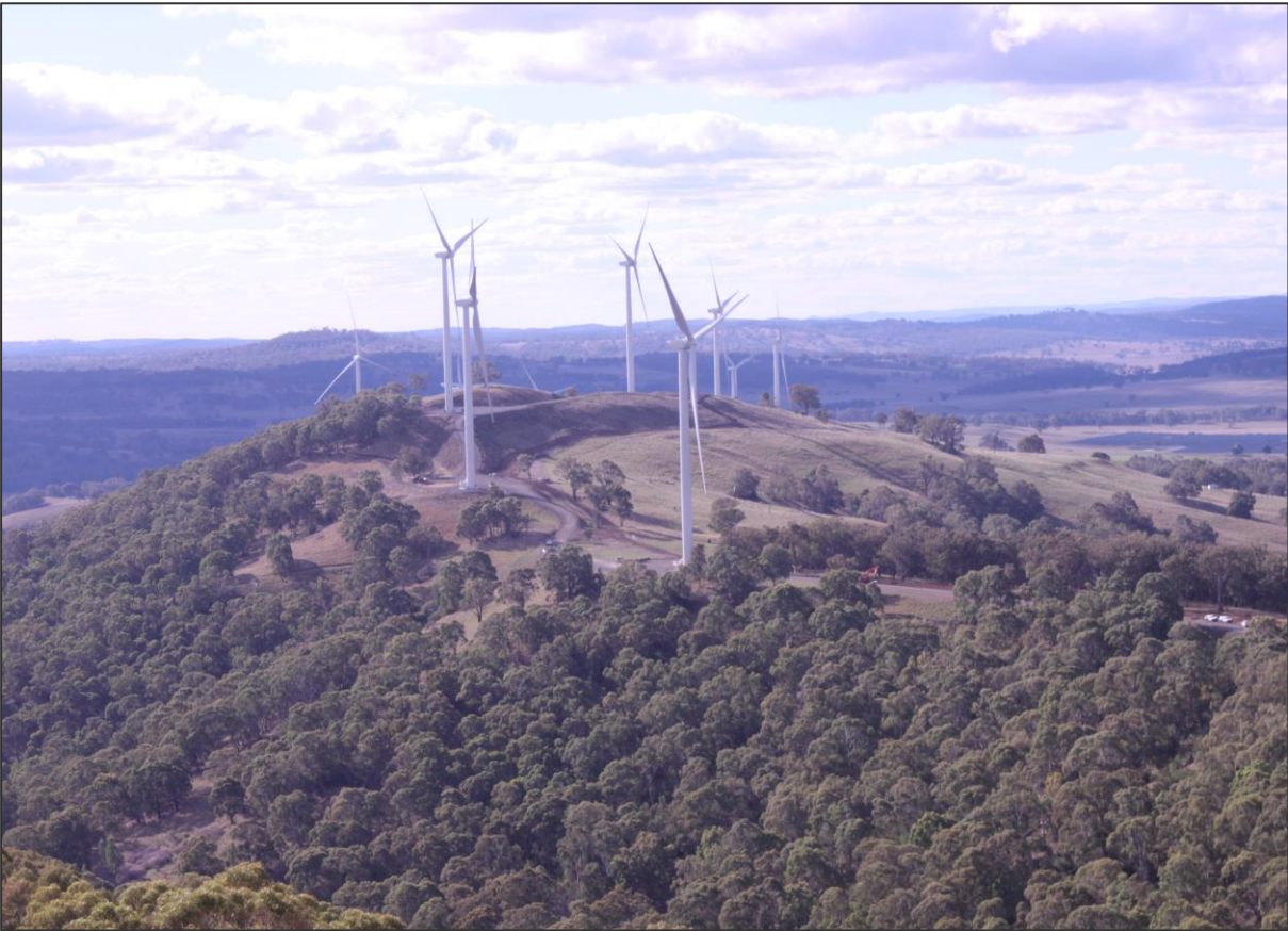
Figure 2 | Photo of constructed Stage 1 turbines
