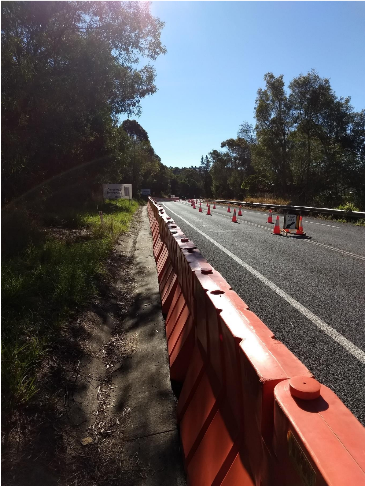
Figure 3 | Gate D approach looking north
