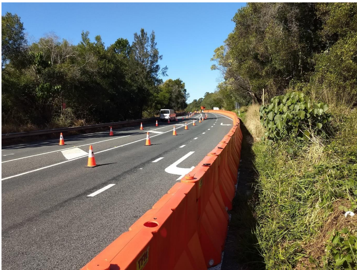
Figure 2 | Gate D channelization, looking south
