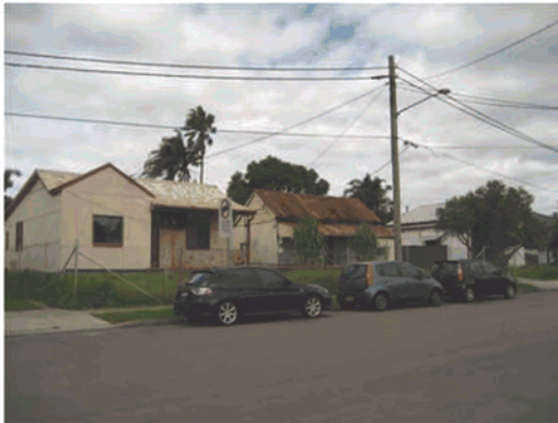
Figure 8 – View of existing development on the site – vacant dry cleaner premises on corner of Silverwater Road and Bligh Street (top left), dwelling houses fronting Silverwater Road (top right) and dwelling houses fronting Grey Street (bottom left)
