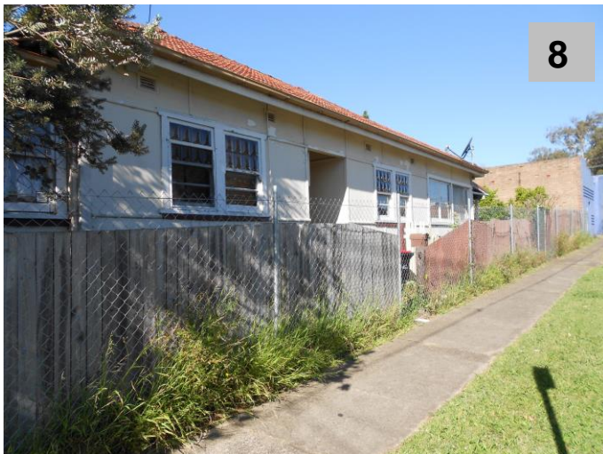
View of buildings on the subject site facing Bligh Street
