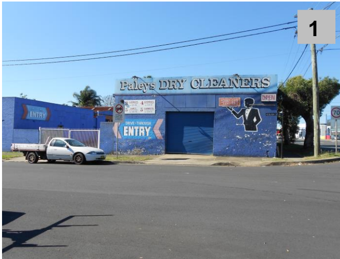
View of the subject site showing buildings facing the corner of Bligh and Silverwater Road
