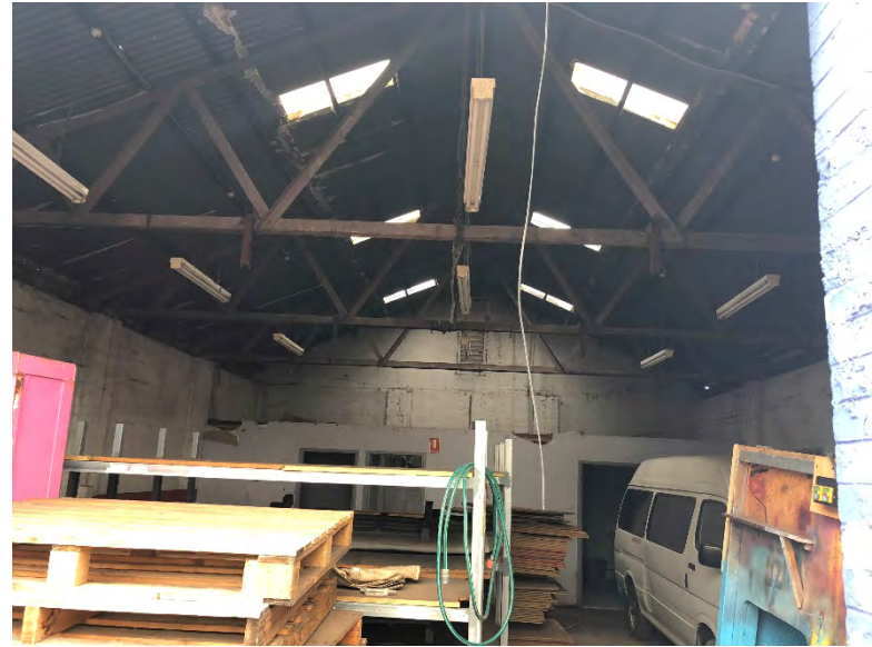
Building C interior – north end.
