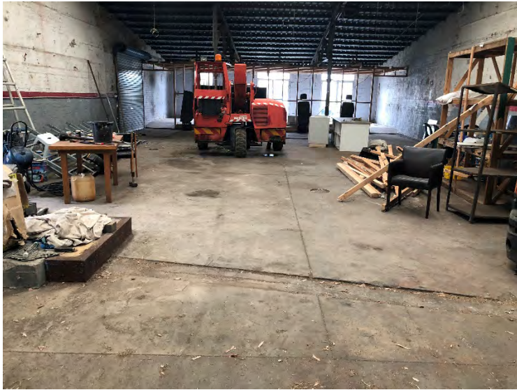
Building A interior – raised plinth and infilled drain and opening.
