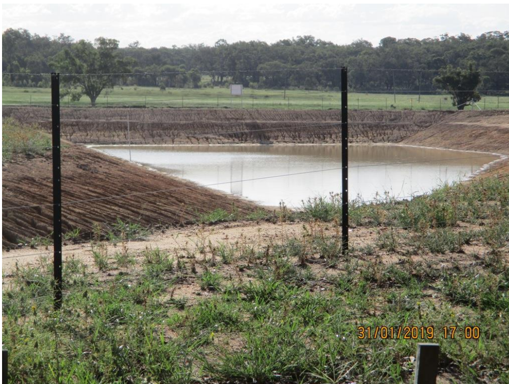
Photo 12. Borrow Pit Dam on Lot 8.( 31.01.2019 )
