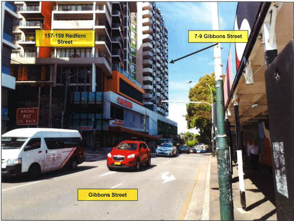
Figure 8 | Redfern Town Centre looking south along Gibbons Street (Base source: Department’s photograph)
