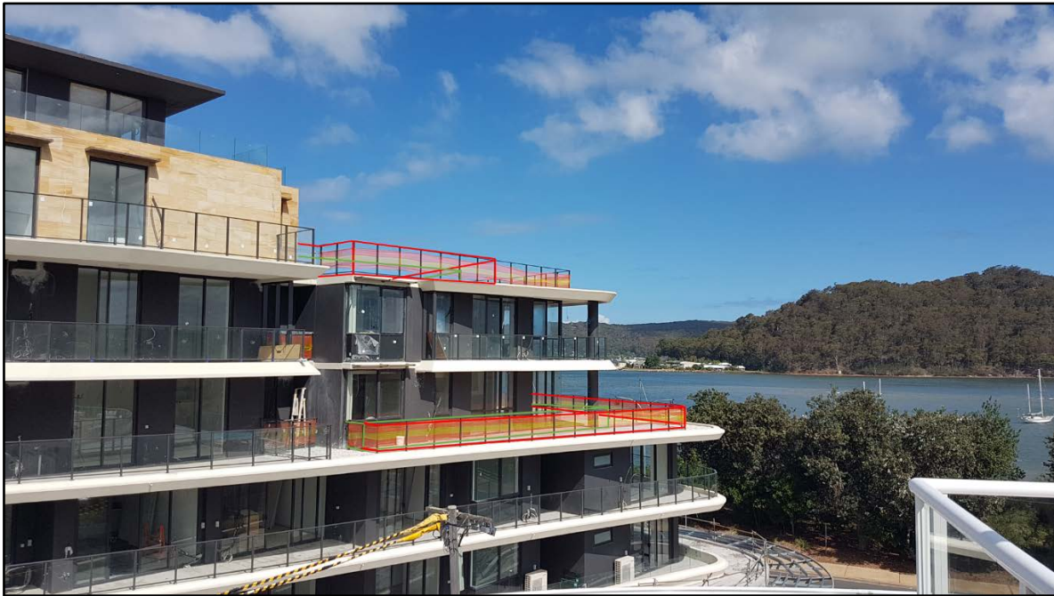
Figure 19: Visual impacts of approved (green) and proposed (red) balustrades from Location A – lower level apartment balcony at the Mantra (Base source: Department’s photograph 29.11.18)
