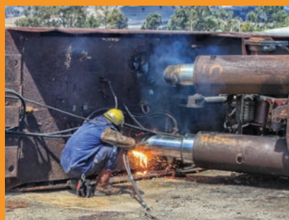
Roof support section being dismantled
