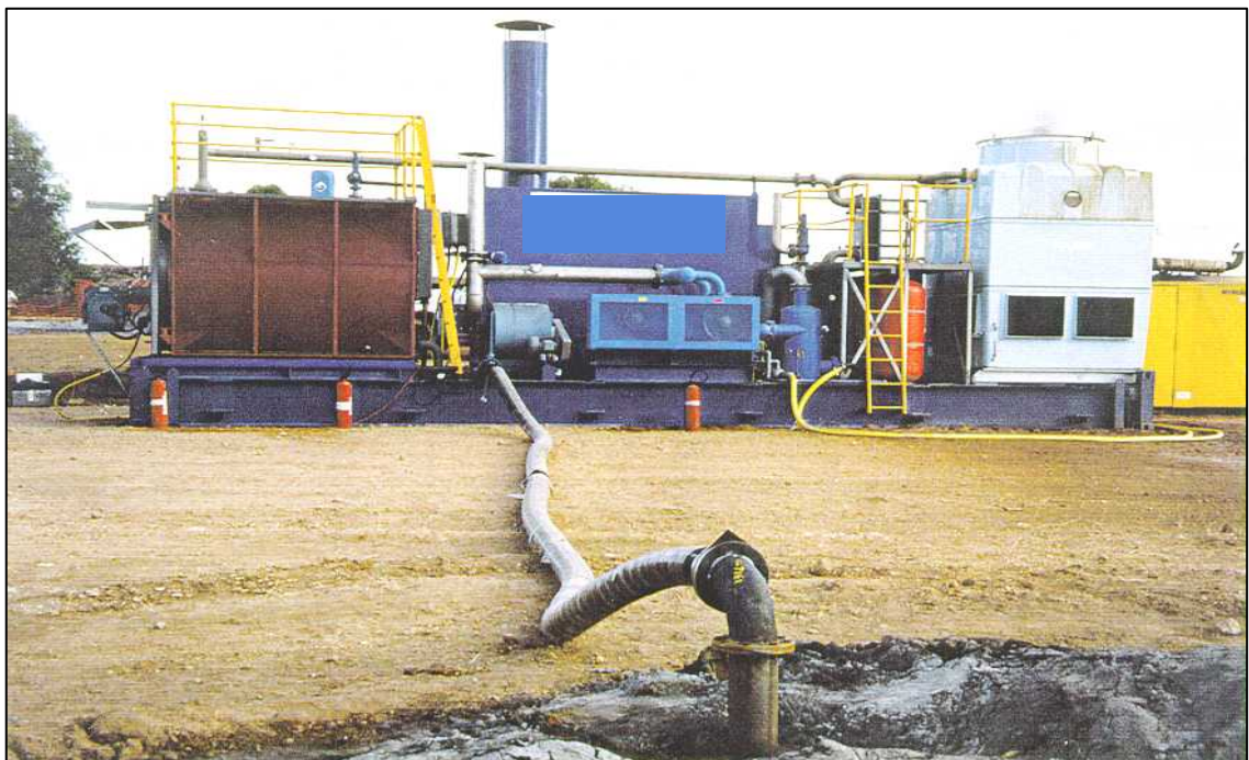
Figure 32: Tomlinson Boiler unit discharging down a borehole
