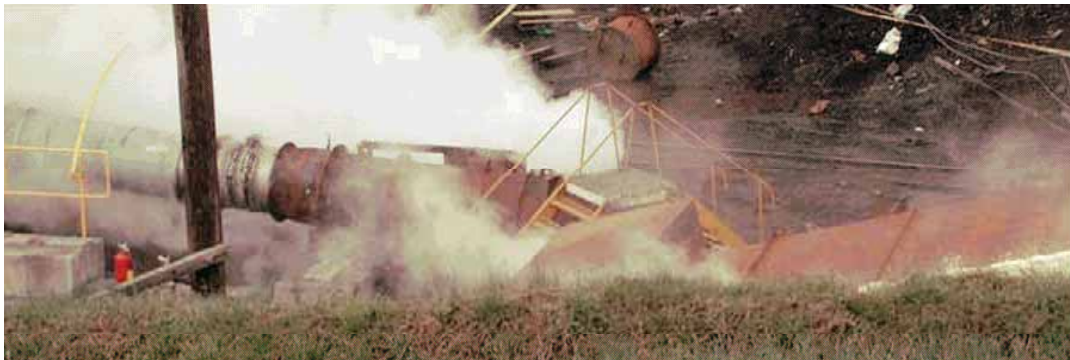
Figure 2.12 GAG 3A jet engine system interface with Sugar Run Slope. Note steam indicating exhaust gas leakage.
