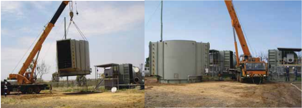
Figure 4.3 Removed Main Fan Dividing Breach on top of shaft.
