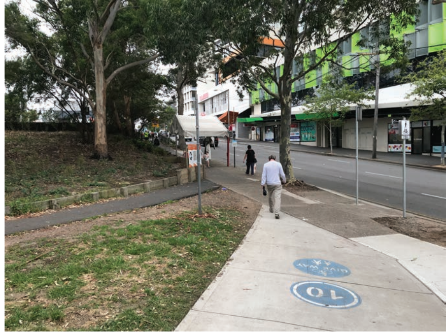
Image 4h. View of path from site to Redfern Station northern entry. Series 4 of 6. Source: Author
