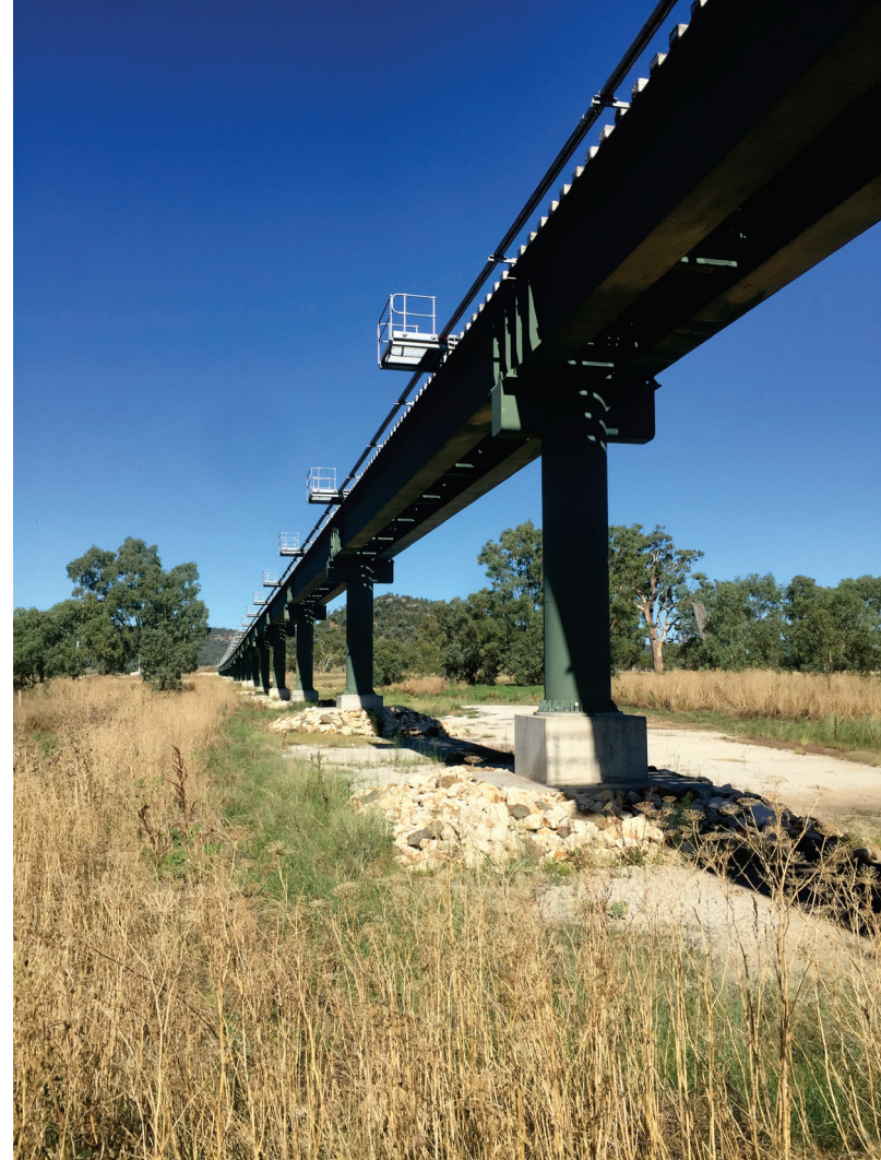
Plate 2b Maules Creek and Boggabri Coal Mine Rail Spur
