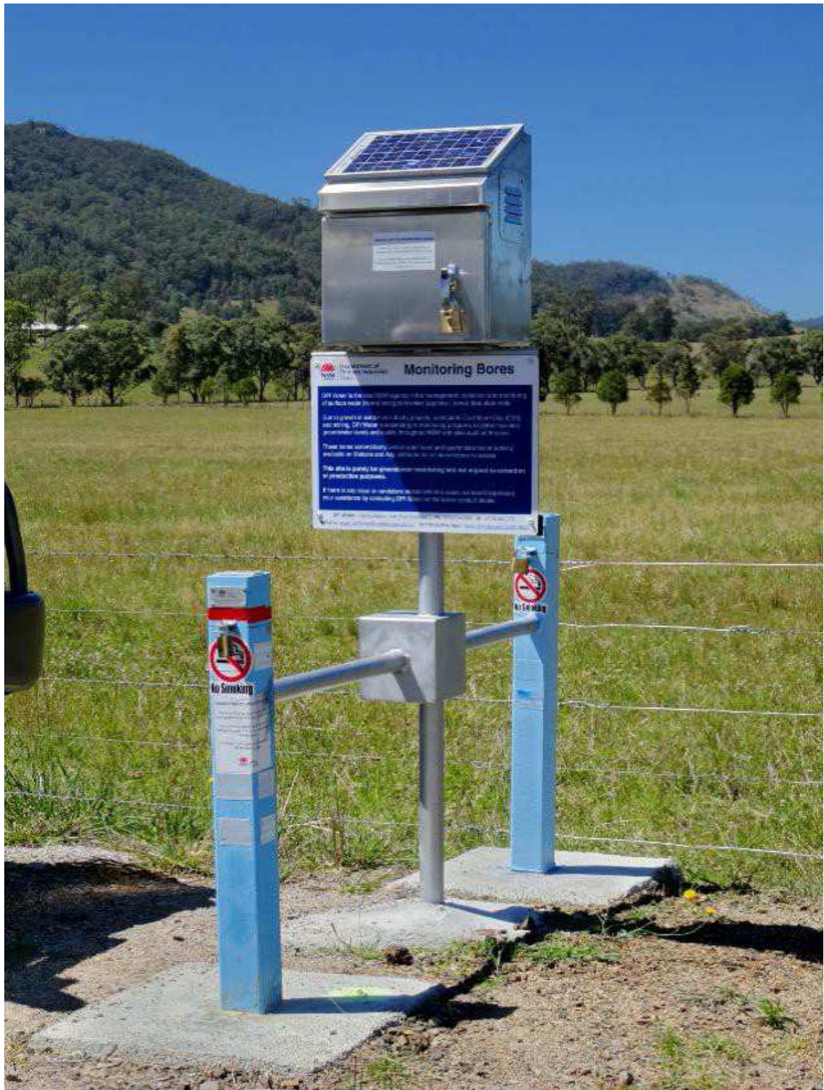
Figure 3-3: Typical site set up for water monitoring bore constructed to Minimum Construction Requirements for Water Bores in Australia
