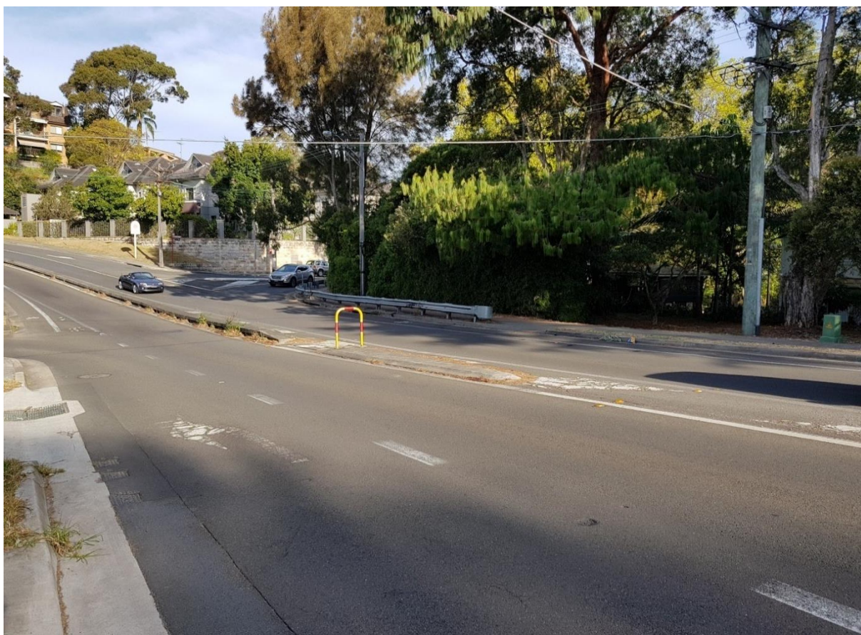
Photograph 2: Existing Refuge Island at River Road and Canberra Avenue Intersection
