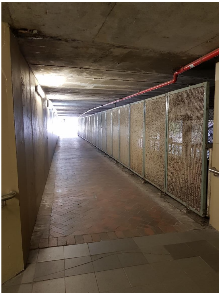
Photograph 1: Existing pedestrian underpass across the Pacific Highway (looking north)
