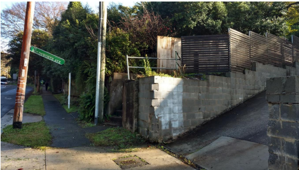
Figure 9 Pedestrian link at the intersection of Holdsworth Avenue and River Road.
