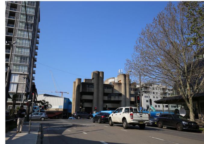
Location 3 - From Oxley Street looking towards Pacific Highway
