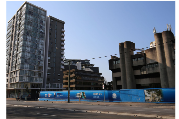
Location 4 - From Pacific Highway looking opposite
