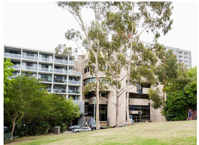
Figure 9- Hume Street Park, looking west towards the Sydney Metro sites
