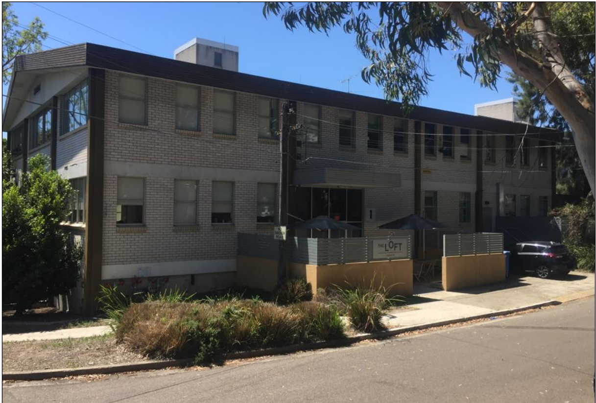
Figure 4 | Existing 'Loft' building and entrance to Scott Street (Source: Department's Photo)
