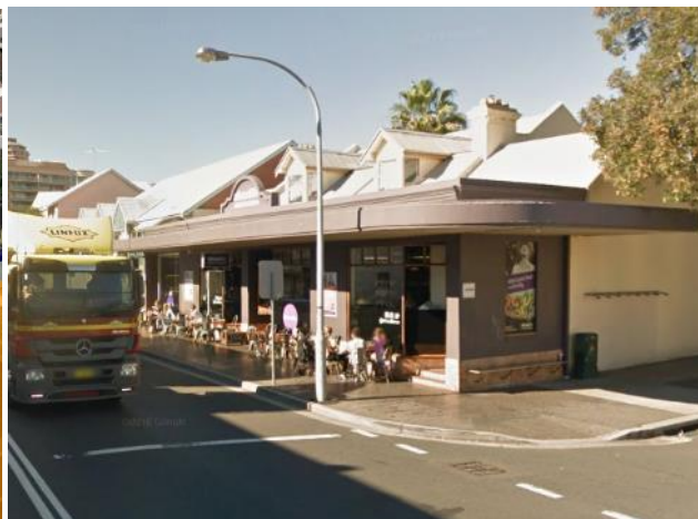
Figure 22: Existing outdoor seating
