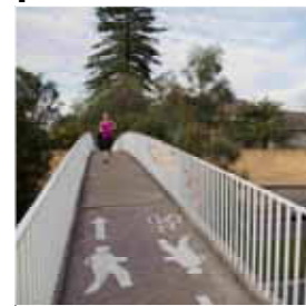
F FOOTBRIDGE OVER FREEWAY
