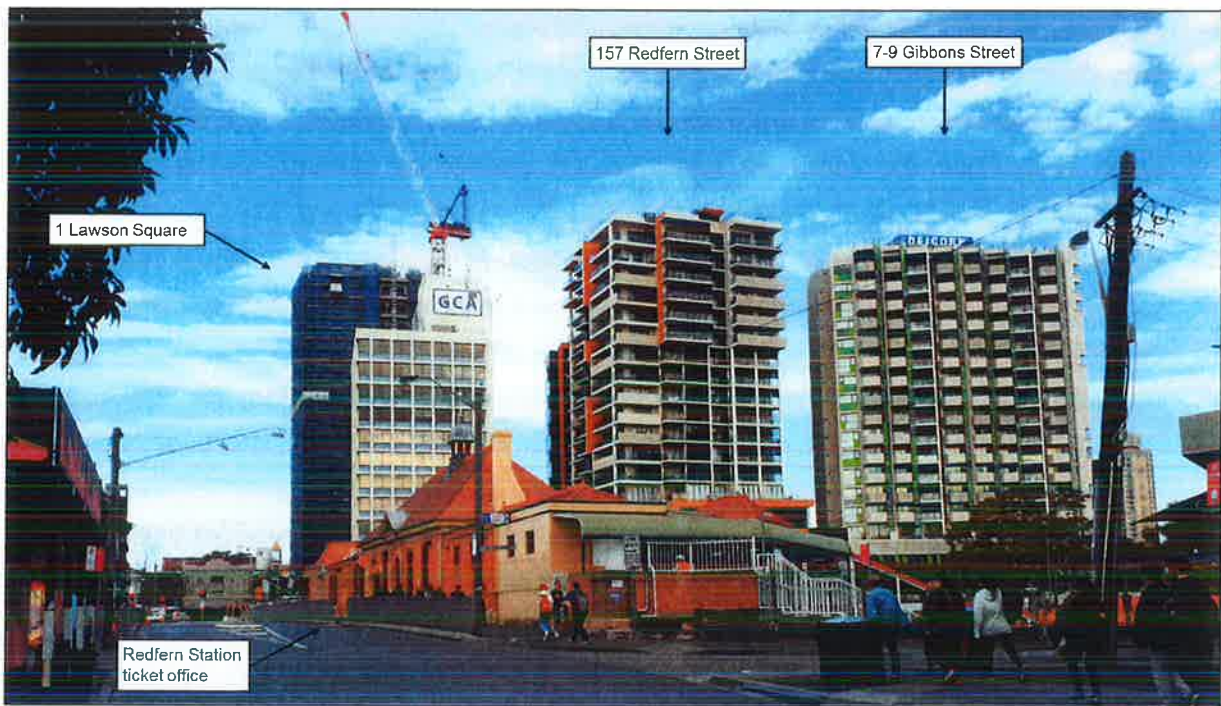
Figure 25 | View looking east along Lawson Street towards Redfern Station and existing towers (Source: Applicant's RTS)
