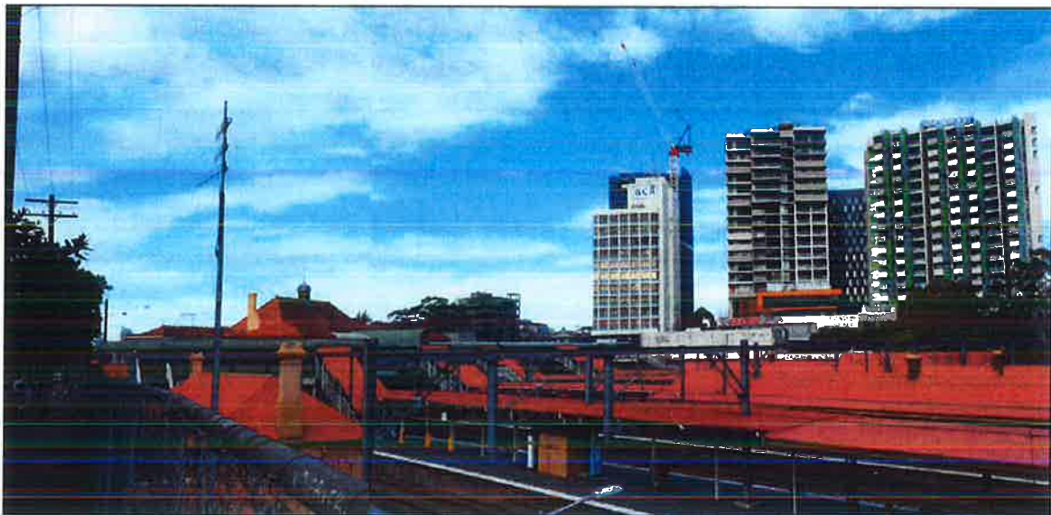
Figure 17 | View north-east from Little Eveleigh Street towards Redfern Station and the existing towers (Source: Department's site visit)
