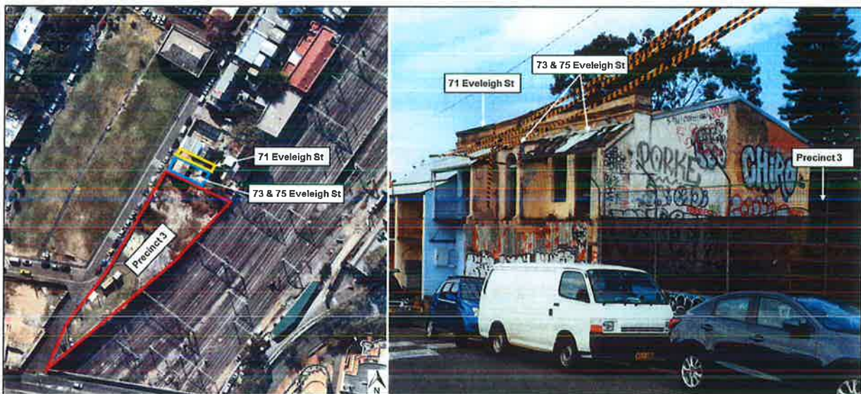
Figure 32 | Location of the closest occupied residential property to the site (71 Eveleigh St, outlined yellow) and adjoining derelict buildings (Base source: Applicant's RtS and Department's site visit)
