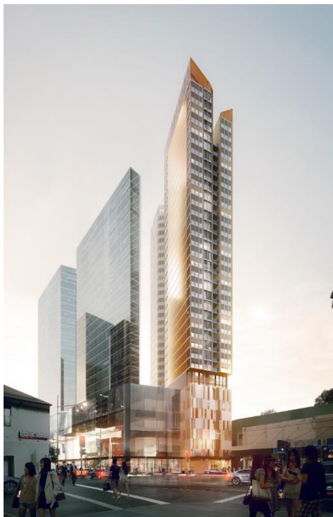
Figure 4 Photo montage of potential built form outcome (55 Aird Street – building to right) under proposed 15:1 FSR without site amalgamation. Blank wall to Church Street allows for future development of adjoining sites that are not amalgamated under this proposal.
