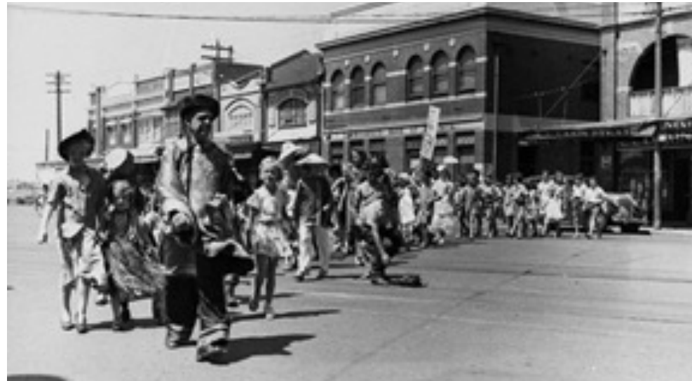
Figure 83: Buildings to the western side of Anzac Parade erected during the Inter War years 1946 Source: www.trove.nla.gov.au
