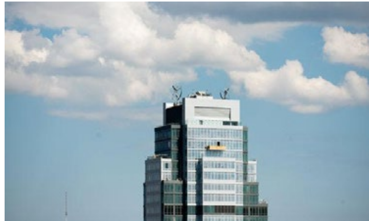
Figure 98: Urban Wind Turbines Source: www.ugei.com
