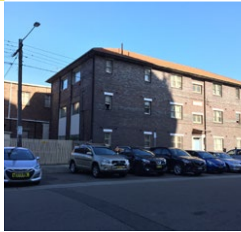
View of existing building at 63 Harbourne Road from Harbourne Road, Kingsford
