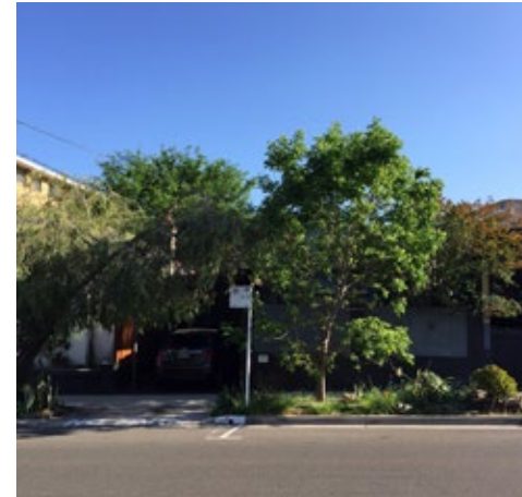
View of existing building on 16 Barker Street from Barker Street
