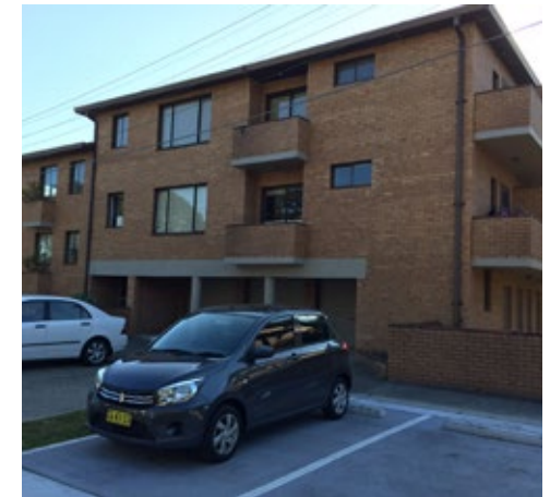
View of existing building at 18 Rainbow Street from Forsyth Street, Kingsford
