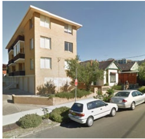
View of existing buildings on subject sites from Barker Street
