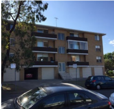
View of existing building on 20 Barker Street from Harbourne Road
