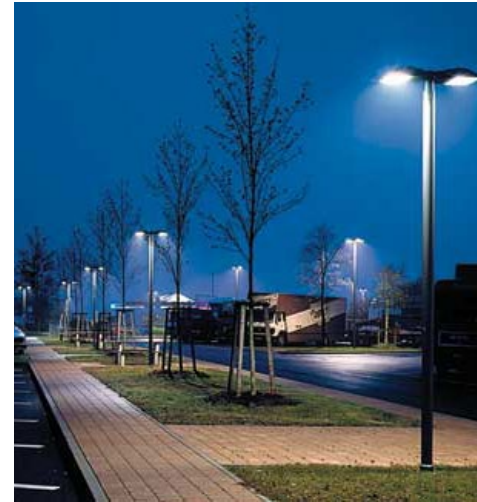
Figure 145: Lighting in public carpark Source: www.usask.com
