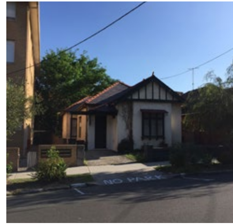
View of existing building on 18 Barker Street from Barker Street
