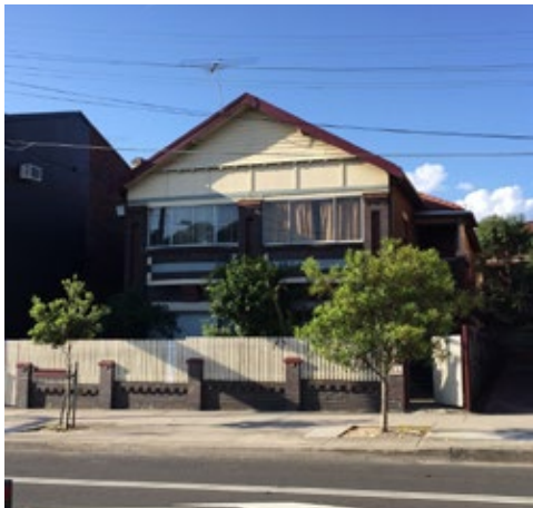
View of existing building at 14 Rainbow Street from Rainbow Street, Kingsford
