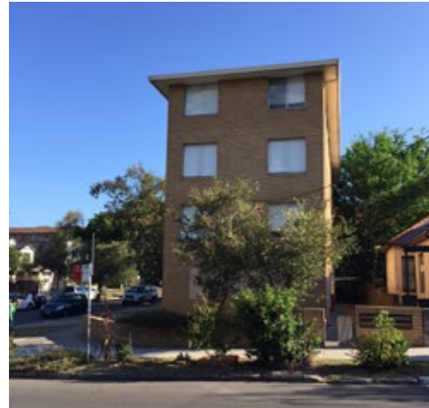
View of existing building on 20 Barker Street from Barker Street
