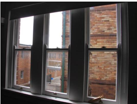
View from living room of east facing lower level unit
