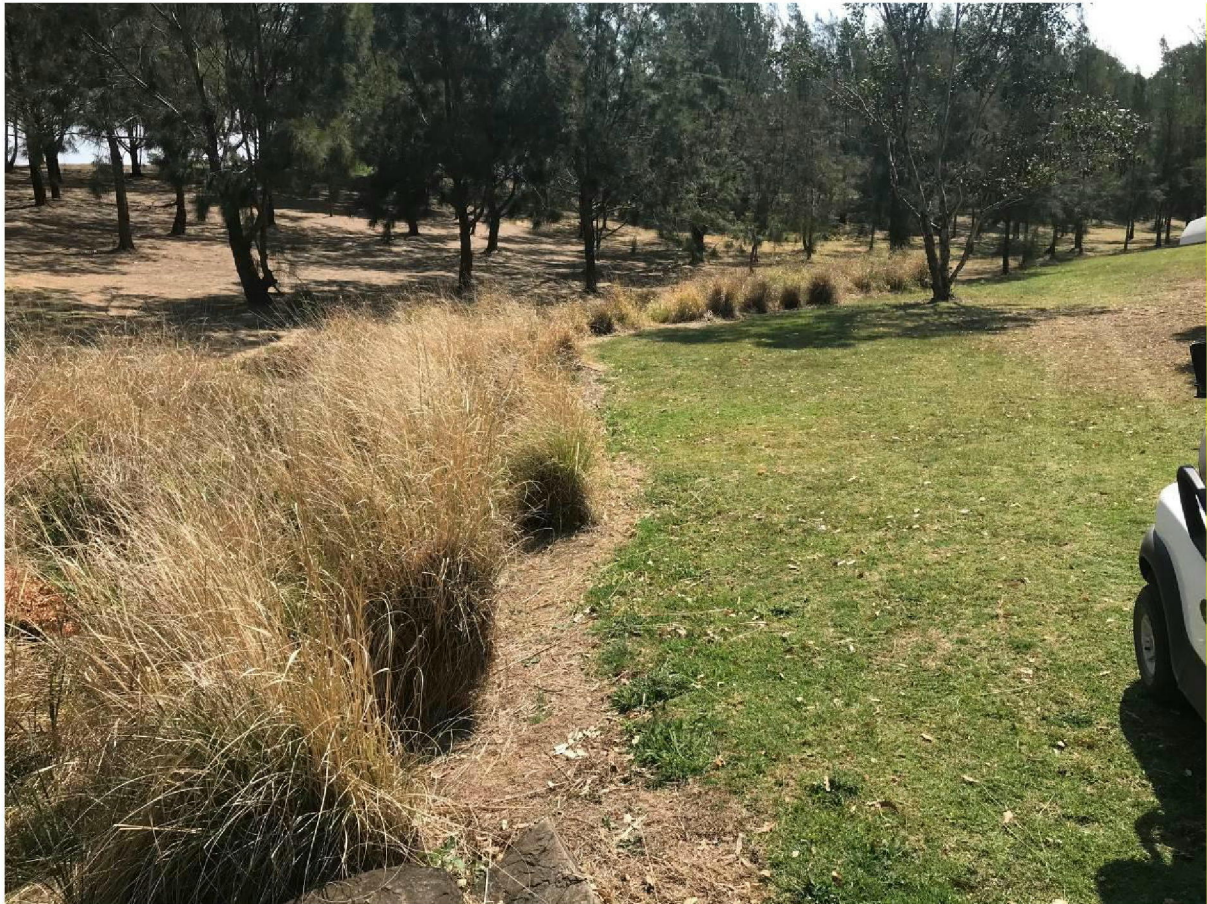
Photo 9 – Watercourse 7 showing existing modified channel upstream of the pipe section
