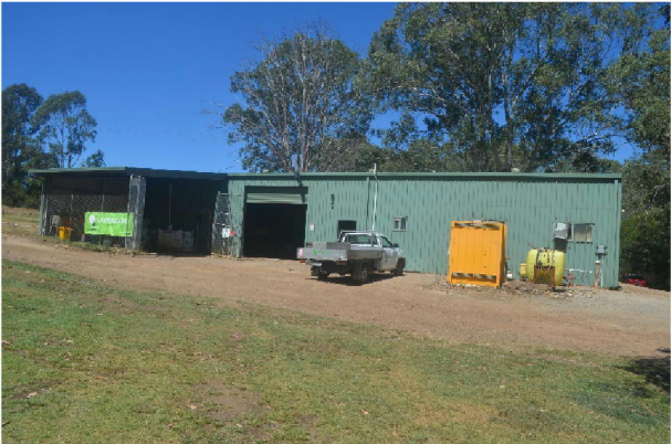
Picture 4 – Existing Maintenance Shed
