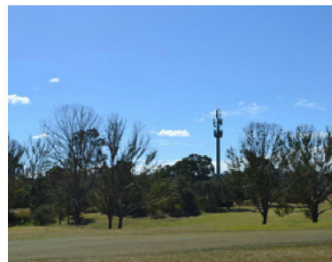
④ Telecom Tower
