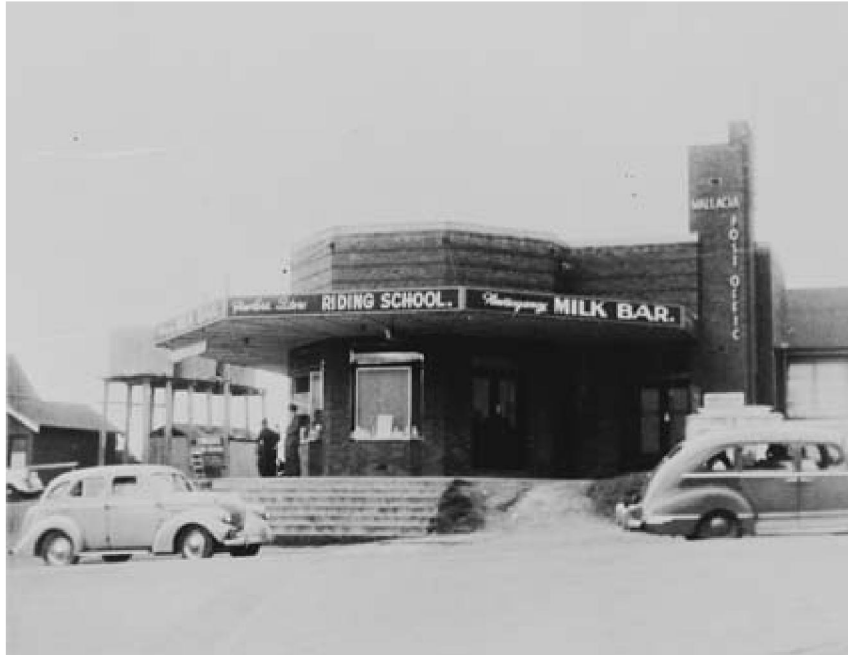
Figure 5.9 Photo of the new Wallacia post office in 1950 (NAA C4076, HN1071).
