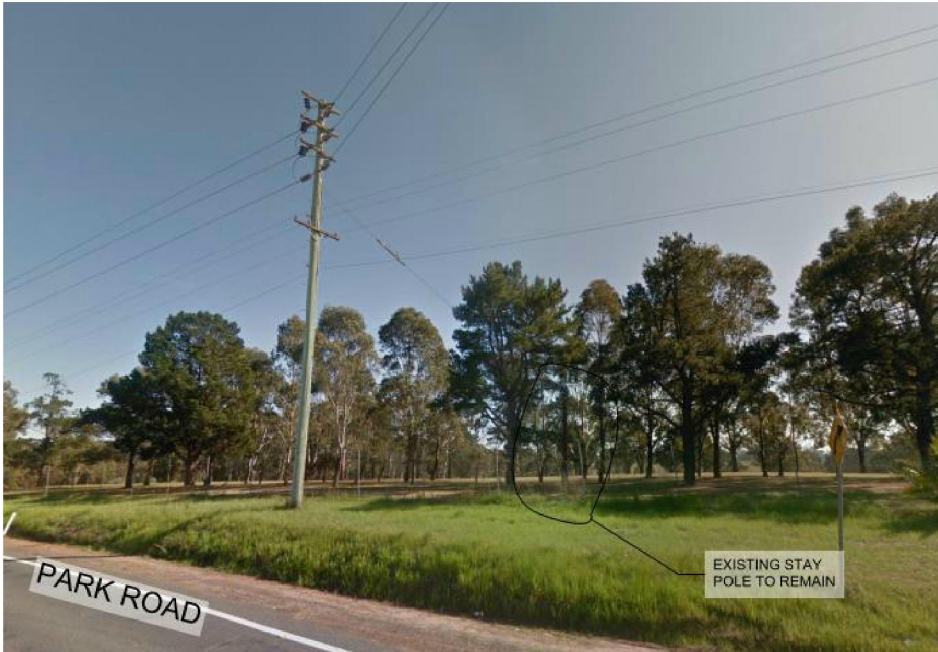
Figure 2 - Existing power stay pole
