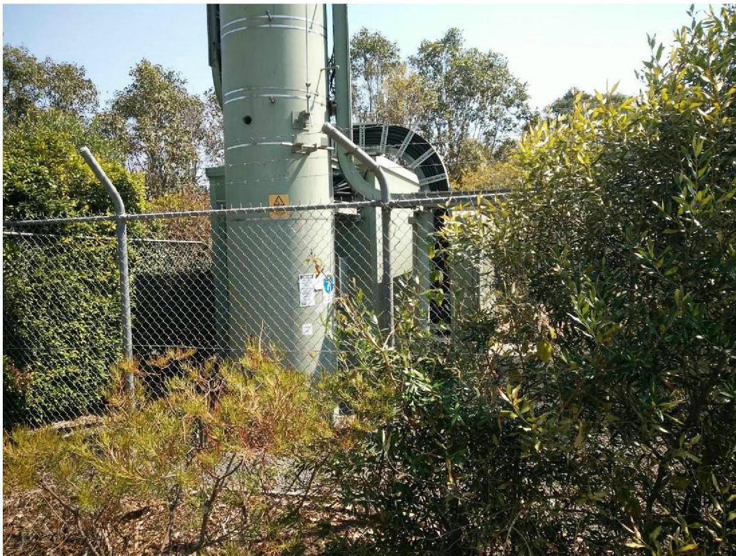
Photo 8 – Planted vegetation adjoining the communications tower.
