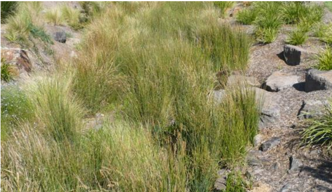
Figure D.1 Typical form of a vegetated swale in Catchment 3 Note the Wallacia SWMP calls for a 1 in 5 vegetated batter
