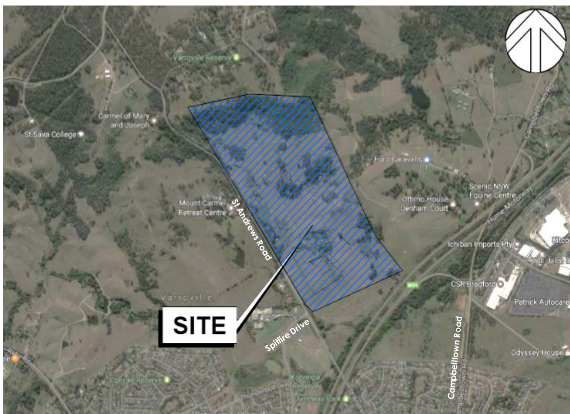
Figure 2.1: Subject Site and Its Surrounding Environs
