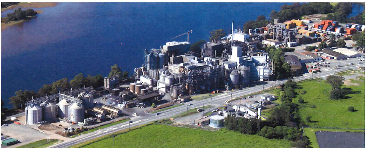
Shoalhaven Starches Factory, Bomaderry
