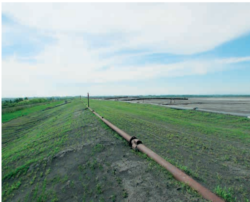
A huge fly ash dumpsite in the vicinity of the Nikola Tesla thermal power plant in Obrenovac, Serbia.
