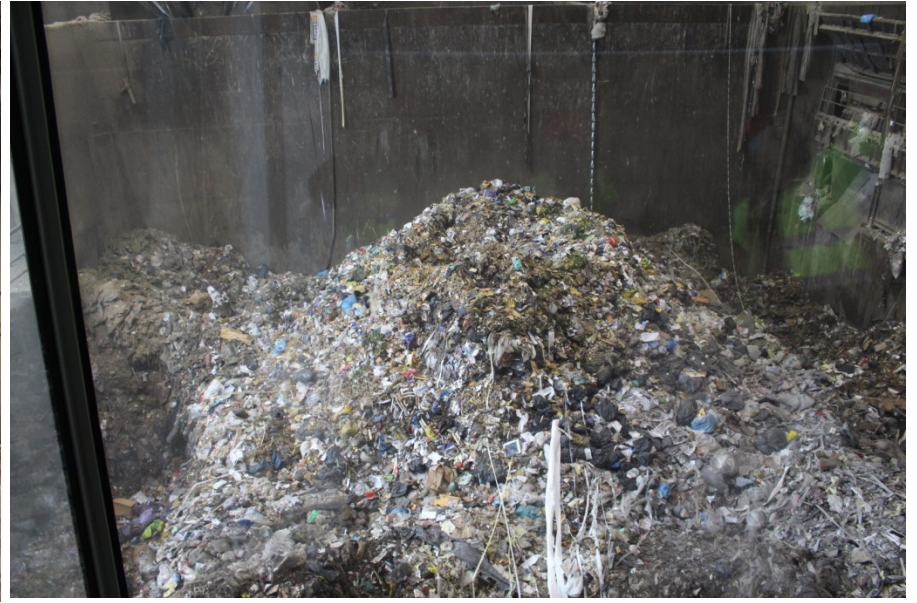
Aarhus Energy from Waste - Denmark
