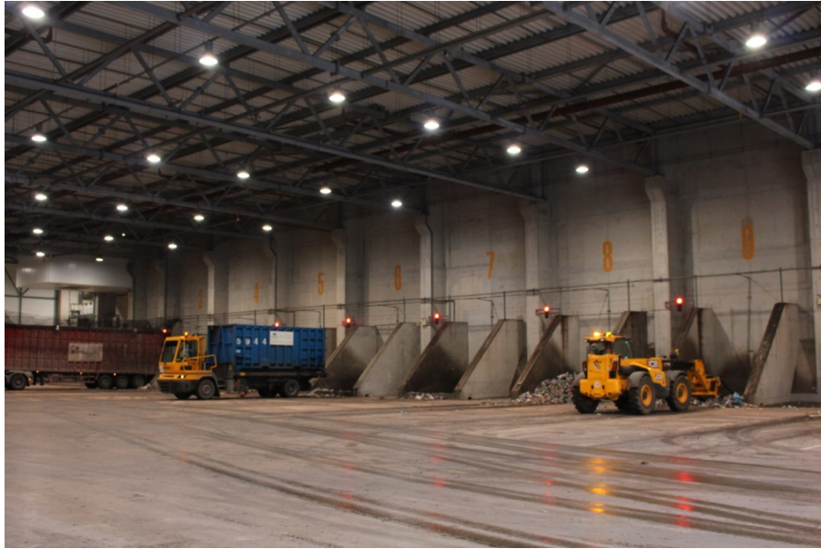
Runcorn Energy from Waste - Manchester
