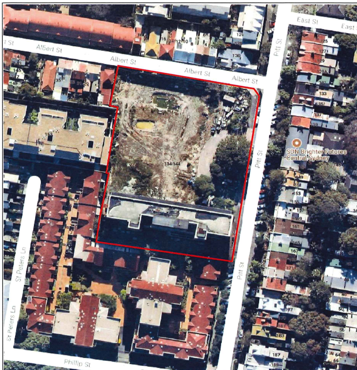
Figure 2: Aerial photo of the site and surrounding locality (site outlined in red) (Base source: Nearmap)
