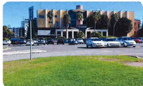
Existing Club and Car Park
