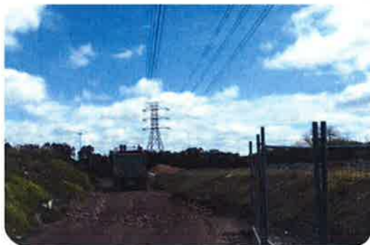
Existing power lines
