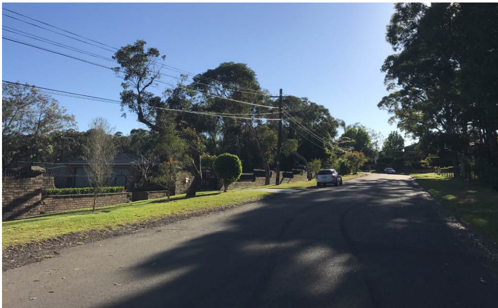
Photo 2 - Looking east along Wyatt Avenue
