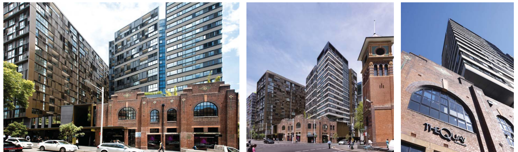
Figure 20 'The Quay', Sydney (WMK Architecture)
