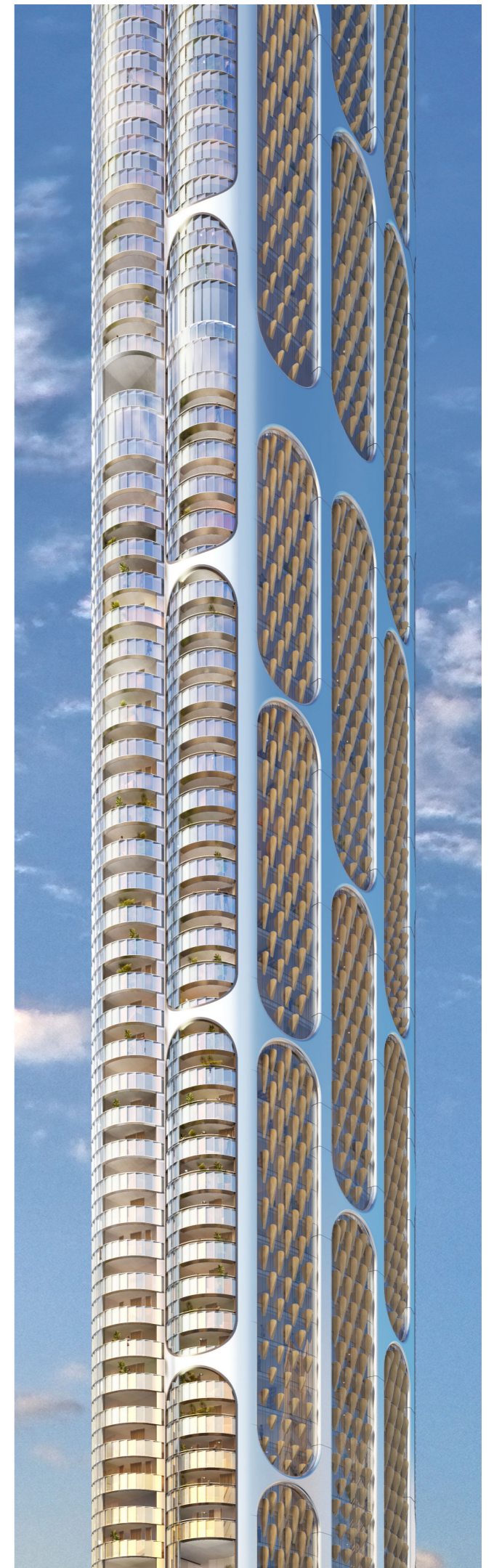
CHURCH STREET VIEW BALCONIES WITH FLAKED GLASS
