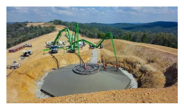
Note that in this photograph there appears to be NIL environmental protection against erosion and sedimentation in place. Additionally note the excavated material stockpiled for re-use (approx. 2000m3). The disturbed area depicted is vastly at variance with that advised by the Proponent for HOGWF in the EIS submissions.
