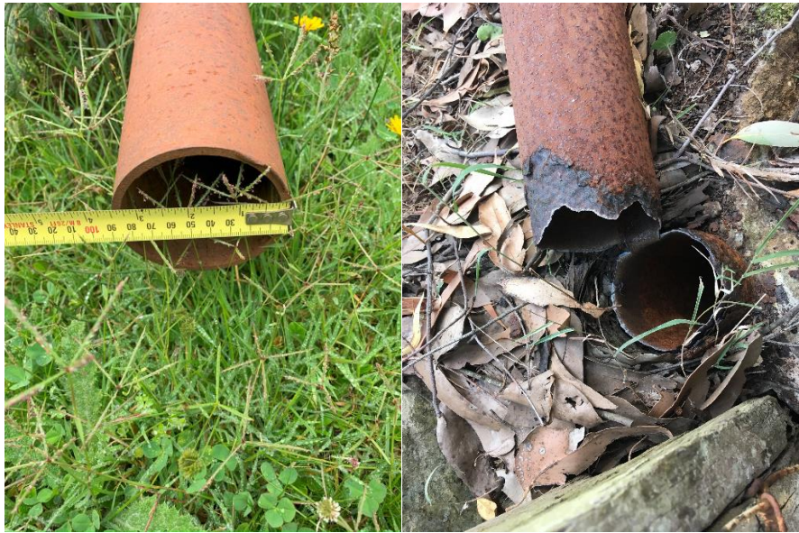
Figure 6: Steel strainer posts.
