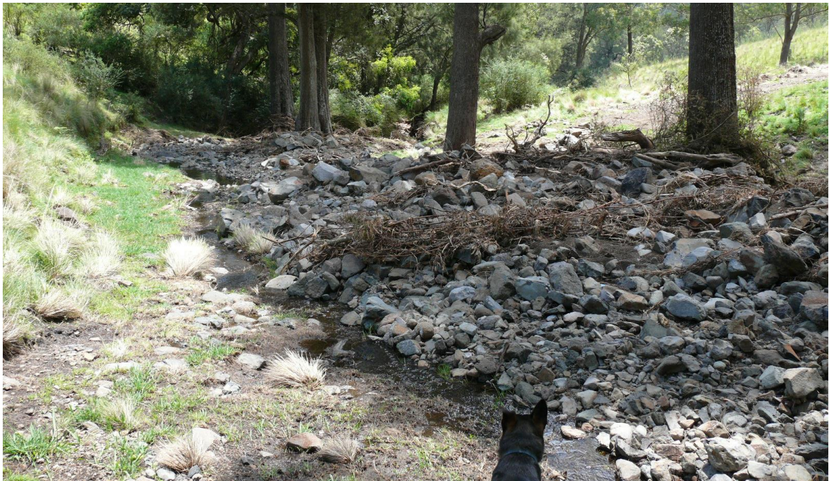
Figure 4: Debris flow deposited during rainfall event of 74mm in 40 minutes, February 2, 2010.
