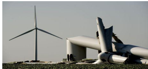
Wind turbine collapse impacts output
