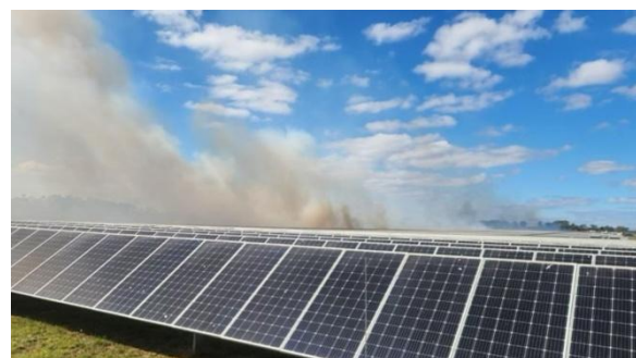
Grass fire burns under the solar panels
