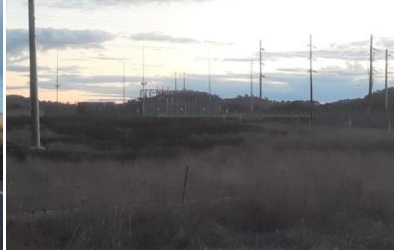
Fire reached solar works fence
